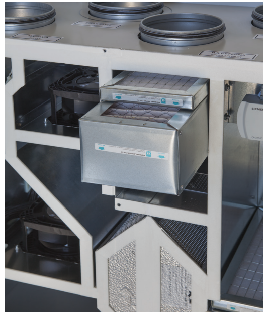
G3 and F7 filters on the supply circuit
