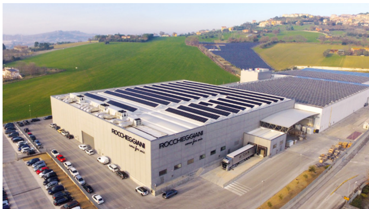
Stabilimento HVAC HVAC department
