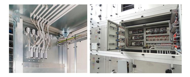
The outputs of the regulators, through the use of transducers, changes the operating parameters of the dampers, the modulating valves, the electric coils, the fans, humidifier, the dehumidifier, the antifreeze system, etc. The regulators can also adapt the air flow or pressure, by means of the microprocessor that regulates the frequency converter changing the number of fan revolutions, according to the set flow rate and the level of filter clogging or air quality.
